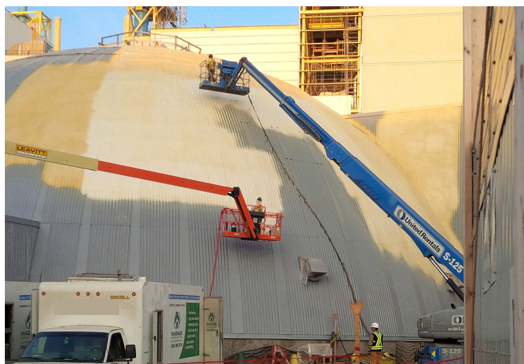
Figure 6. The application of spray-on insulation and top coat.
