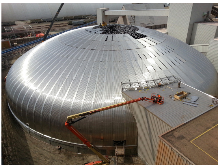
Figure 3. A 73 m (239 ft) dia. steel dome during construction.
