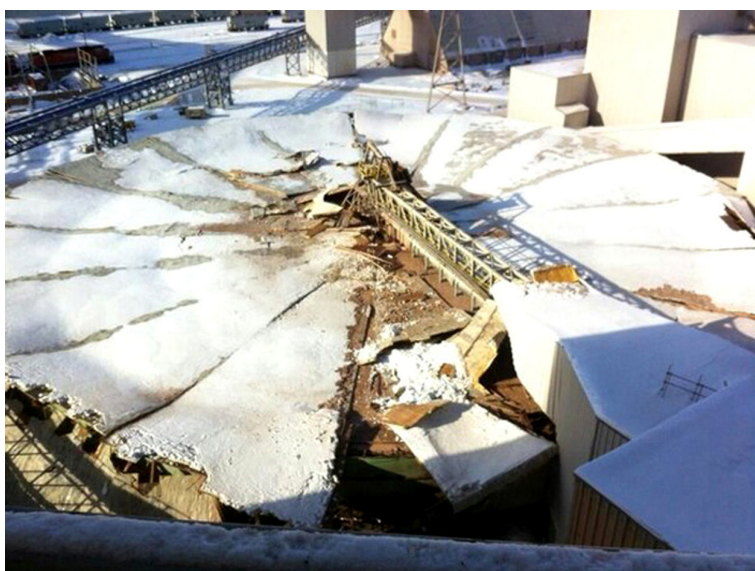
Figure 2. A collapsed timber dome.
