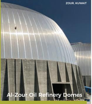
The oil refinery is located on the Persian Gulf. The Port Facility Project consisted of two 88m diameter aluminum domes. Aluminum was chosen because of the corrosiveness of sulfur.
