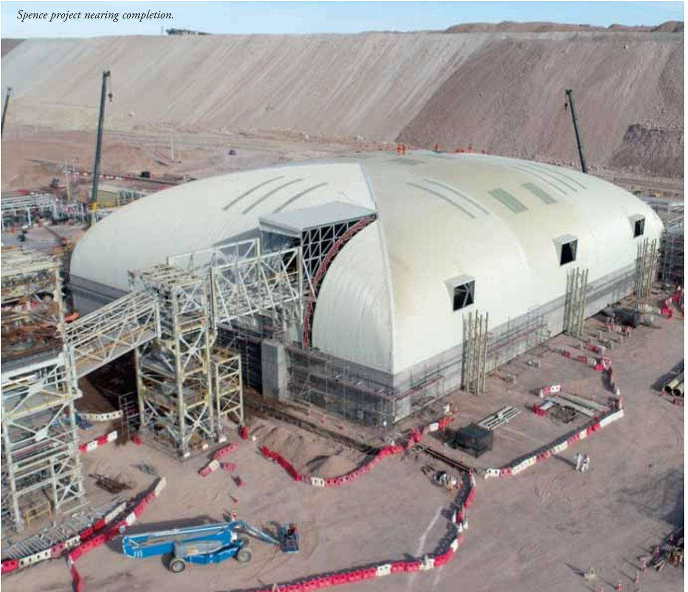
northern Chile, Triodetic was contracted to build two stockpile covers. A rectangular shaped dome cover with major dimensions of 60m by 80m for copper concentrate and molybdenum and a coarse ore dome stock pile cover with a diameter of 110m. First production of 185ktpa (kilo tonnes per annum) of copper concentrate and 4ktpa of molybdenum will be in 2021. As of January 2020 the rectangular dome is completed and the spherical dome is under construction.
